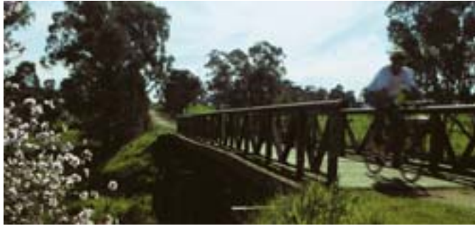
Original Rail Bridge, Strickland Rd
